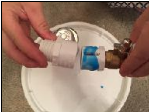
Figure 9 Wipe excess of cement away
