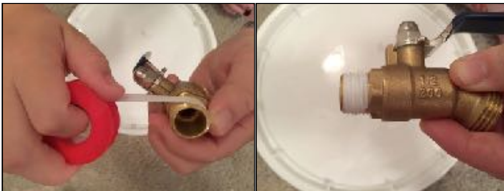
Figure 3 Wrap the male threads of the hose bibb.
