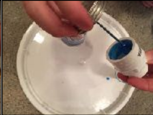
Figure 8 Apply cement to outside bushing
