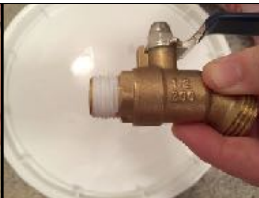
Figure 4 Male threads of a hose bibb taped.
