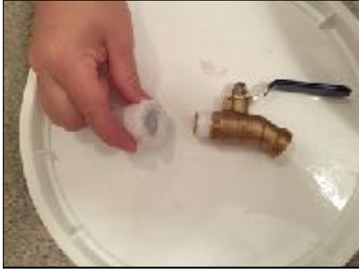
Figure 5 The bushing and the taped hose bibb.
